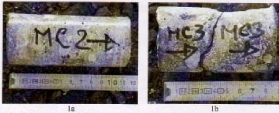
Figure 1. Concrete cored from an undamaged beam (left). Concrete cored from a beam exposed to fire (right)
